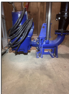
Inside Wet Well – Sump Pump
